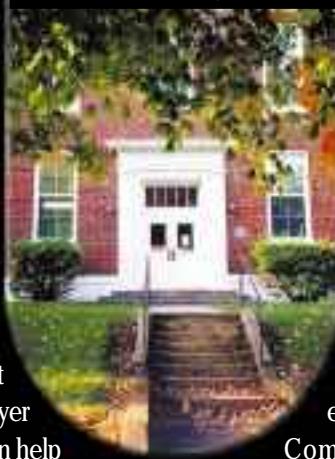
Historic Dickson County Courthouse
